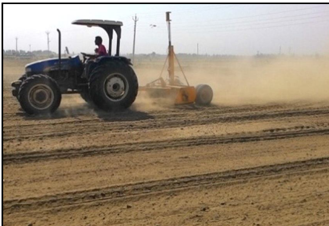
Fig. 1: NSS/GPS-based topographic surveying and land levelling system.
